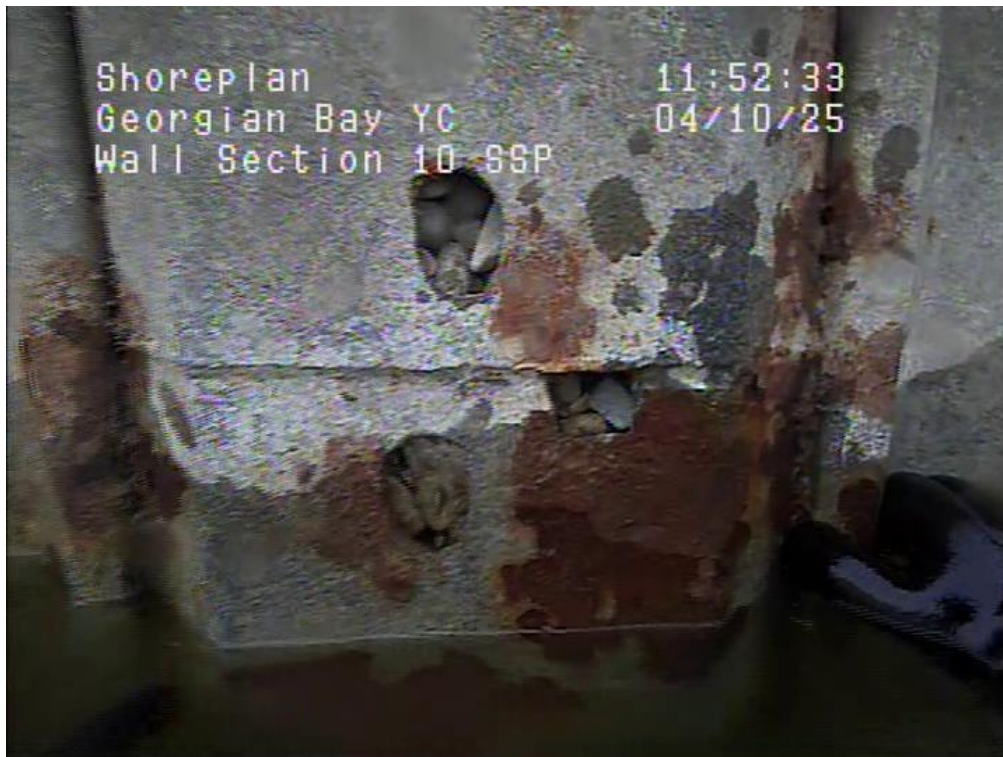
Photo 3.27 Weld Seam and Lift Holes in SSP (10/04/2025)
