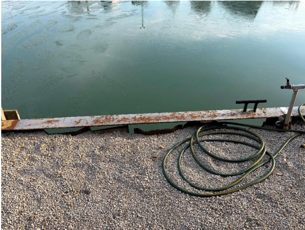
Photo 3.18 Splitting of SSP Knuckles (10/04/2025)
