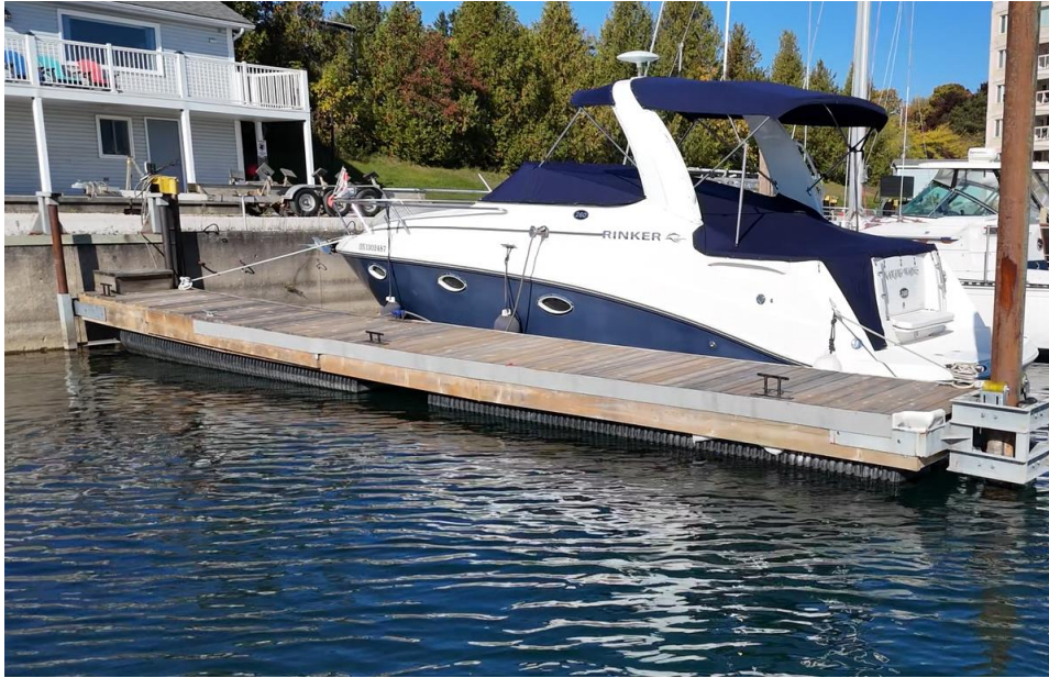
Photo 5.3 View of Floating Dock with Pile Anchor
