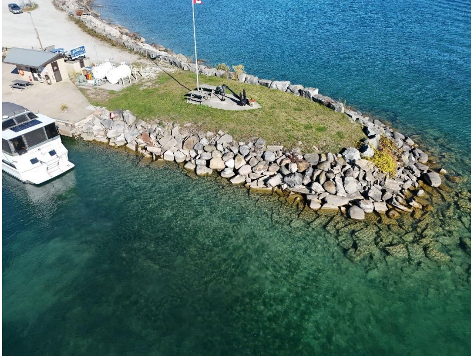
Photo 4.3 View of South Side of North Breakwater (2024 10 18)
