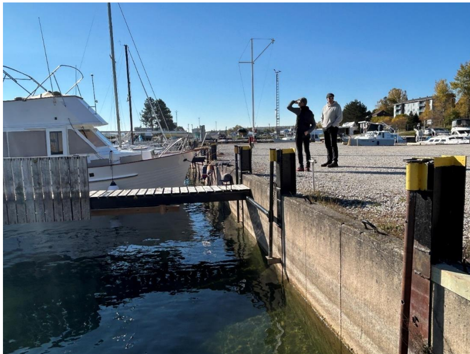
Photo 5.2 View of Fixed Dock Wall Connection
