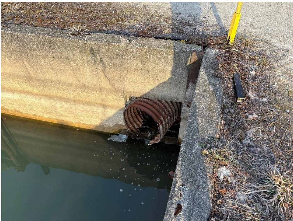
Photo 3.19 Pipe Outlet at S12 (10/04/2025)
