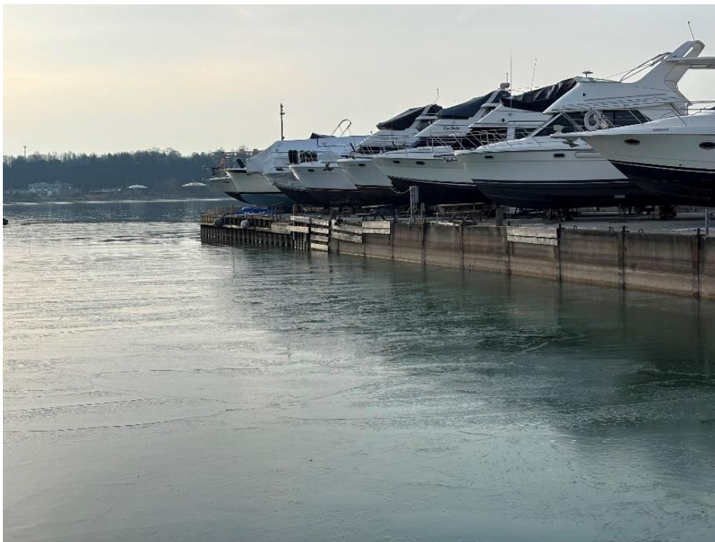
Photo 3.8 Entrance Area South (10/04/2025)
