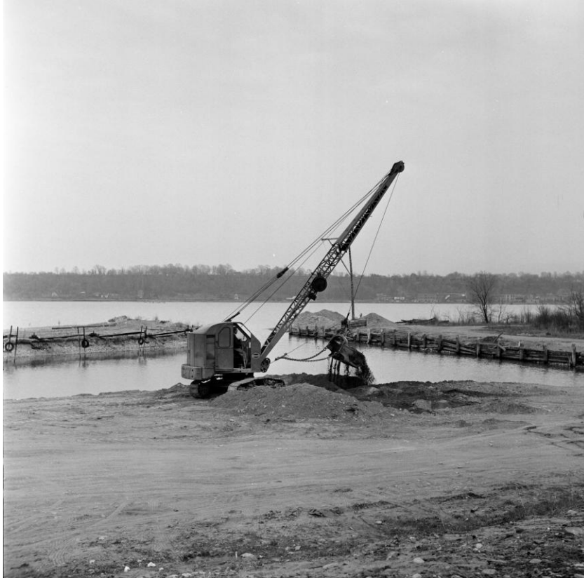
Figure 5: Dragline dredging the north and west basins in 1957 (G. McDonald) [4]
