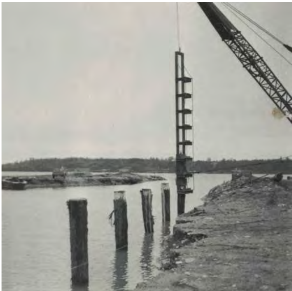
Driving piles along the southern edge of the first basins, circa 1955
